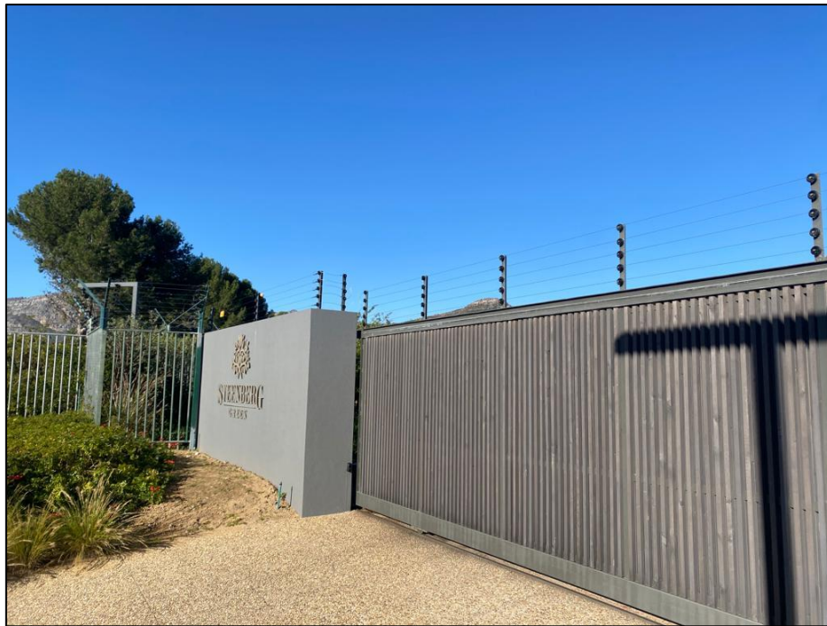
Figure 10. Steenberg Green Main Gate – Advice on how to modify the existing electric fence was provided. This will assist in preventing baboon access.
